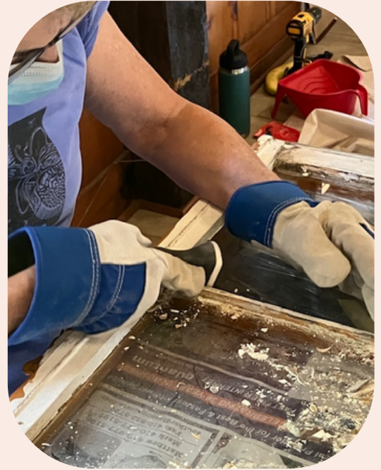
Carefully Removing Glaze Putty
