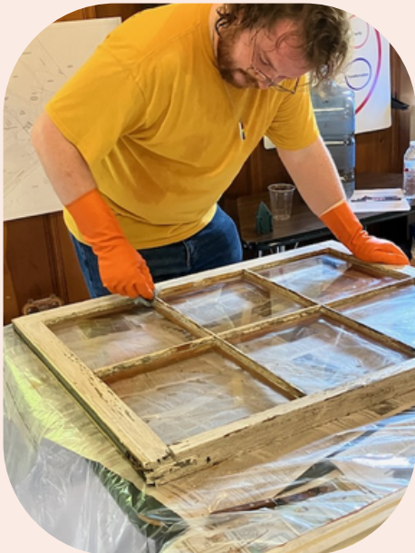
Applying a Wood Preservative Before the Primer Paints are Applied
