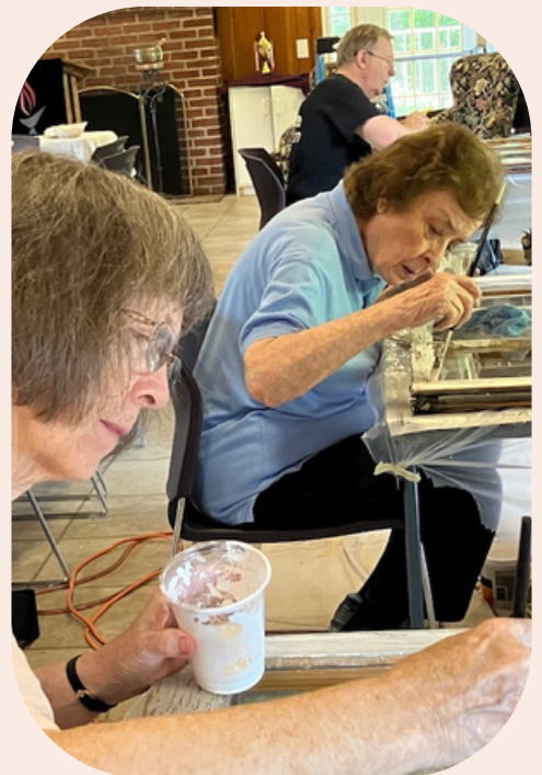
Applying Primer Paint to the Windows
