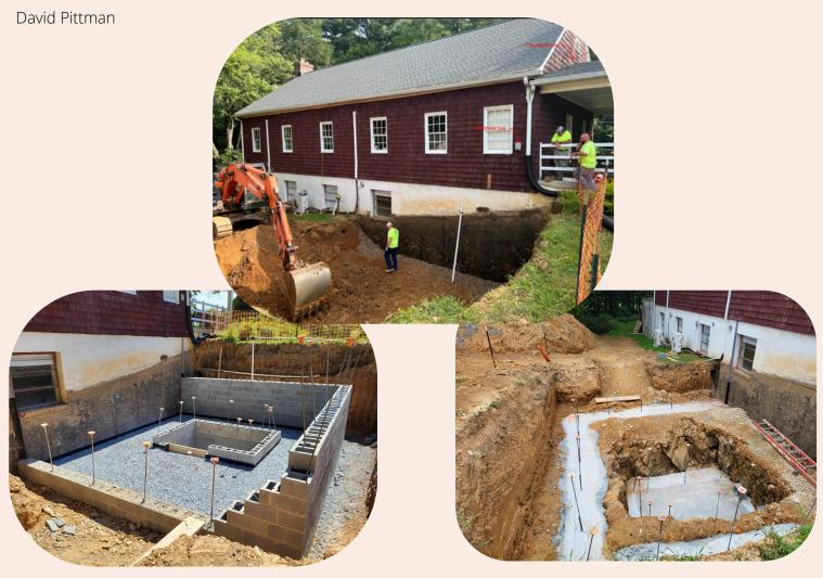
The depress in the center is for the elevator shaft.
